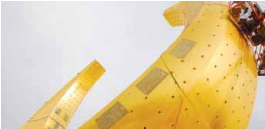
The clock tower includes 23m carbon clock hands and the 23m self-supporting carbon Hilal (above).
