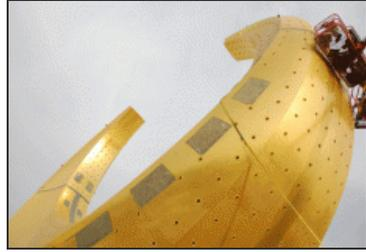
The clock tower will have a 23m self-supporting carbon Hilal.
